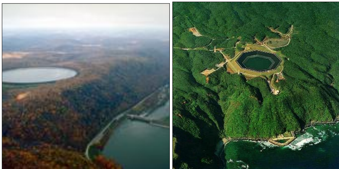
Figure 4.11. Pumped hydro energy storage stations in (a) Pennsylvania – USA (source: Margaret Luzier, U.S. Army Corps of Engineers) and (b) Okinawa - Japan (source: Agency of Natural Resources and Energy Japan)
